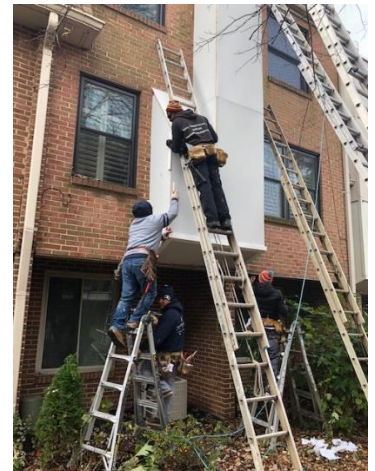
1655 Kenwood Avenue: A new chimney box nears completion
