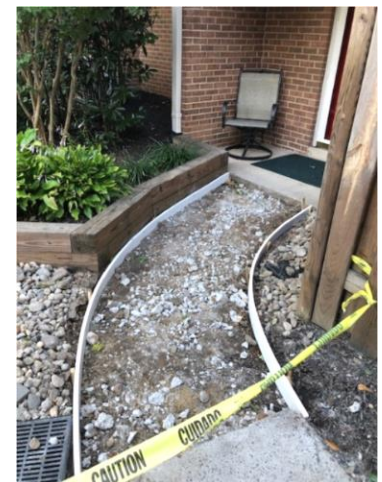
New sidewalk under construction at 1724 Dogwood Drive
