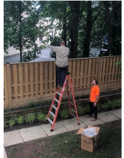
Dominion contractors repairing a neighborhood watch light by 1768 Dogwood Drive.
