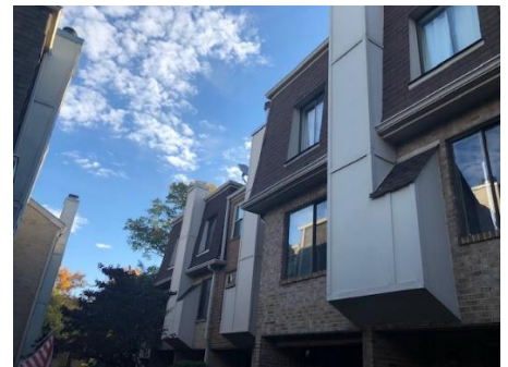
Three new chimney boxes serving 1627, 1629, and 1631 Kenwood Avenue
