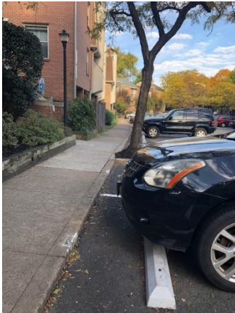
Wheel tops preventing vehicle intrusion
