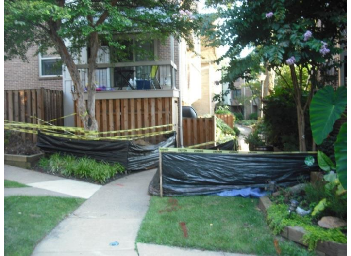
Areas initially excavated following a new electrical outage.
