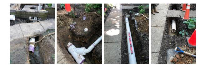
The project started by digging up a trench to the side near 1776 Dogwood Drive to put the trunk line and downspout drains. All other units affected were separately informed of the upcoming work and impacts. Additional pictures below showing the installation work of the new PVC line as per the scope of work.
