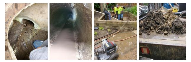
The contractor was able to flush the clogged pipe as shown in the pictures above. Everything was completed in a timely fashion. Work on the stormwater drainage continued with no further complications.
